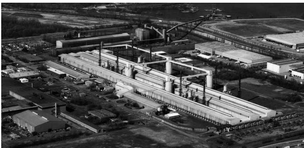
TRIMET plant in Hamburg: electrolysis and anode factory
